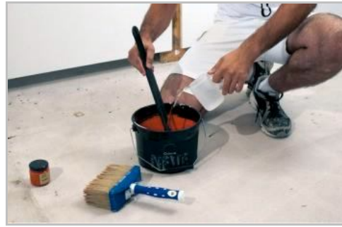
Step 2 - Prepare the shade with Neve and add 30% water solution.
