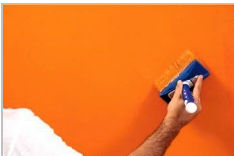
Step 5 - Second coat by "pull and blend"
