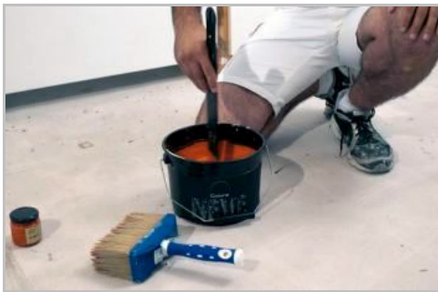
Step 3 - Mix the product until it's homogeneous
