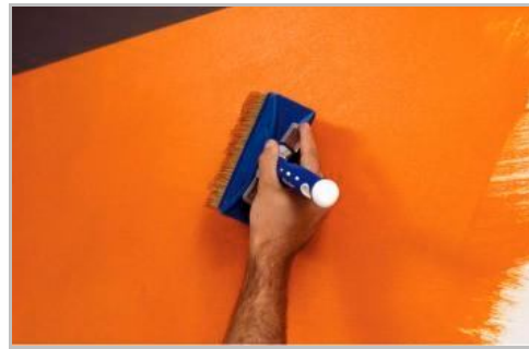
Step 4 - First coat by "pull and blend"
